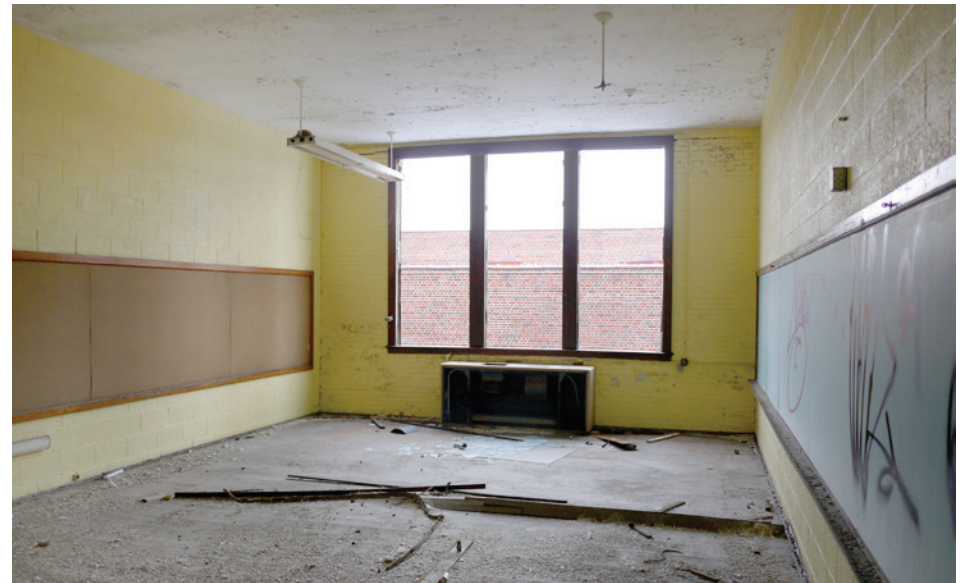
A classroom on the mezzanine level above the gym. This space was likely a second-floor playroom with the same footprint as the gym below, but was later divided into three to create additional classroom space..
