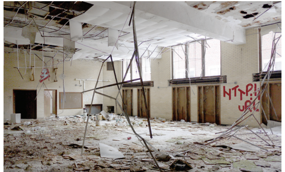
Water damage above the gym has caused the ceiling to collapse. There are three classrooms above this gym.
