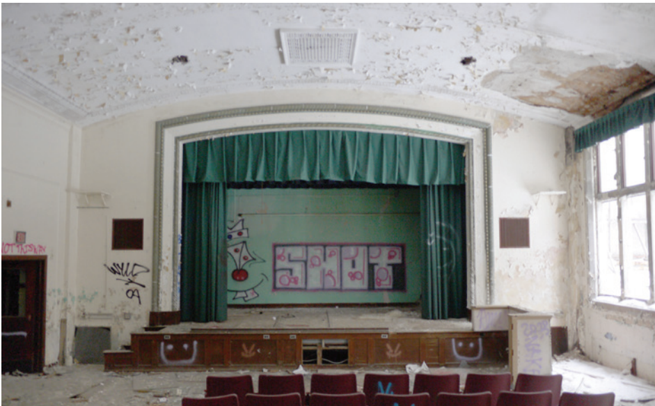
The auditorium features a suspended barrel-vaulted ceiling.
