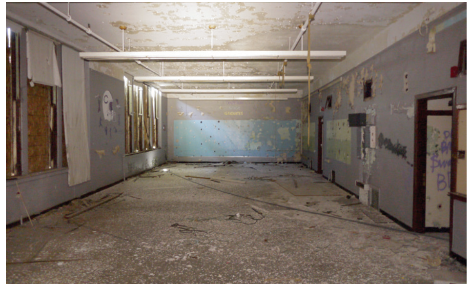
As a former vocational school, Crockett has a number of double-length classroom spaces that were used as workshops and training rooms. On the first floor, many of these large rooms also have extra-thick wood floors, meant to stand up to operating machinery and heavy wear and tear.
