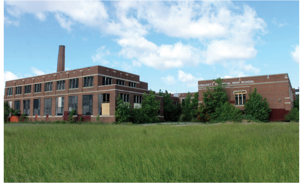
Exterior viewed from the rear (east elevation). The 3-story structure to the left houses the gymnasiums and cafeteria. The 2-story classroom wing is visible on the right. The photo is taken from the adjacent City-owned parcel that was formerly a public park.
