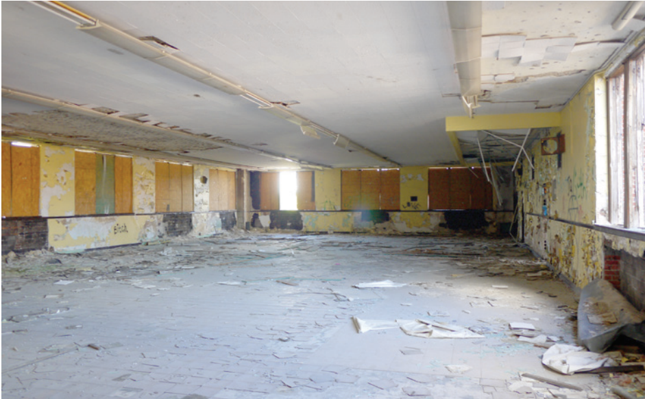
A cafeteria with a large dedicated kitchen sits on top of the two gymnasiums. With windows on all four elevations, this space would have been brightly lit and with sweeping views of the school and adjacent park.
