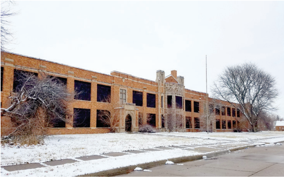
View of the front (south) elevation from Elmira St. The majority of classrooms are arranged along the south elevation.
