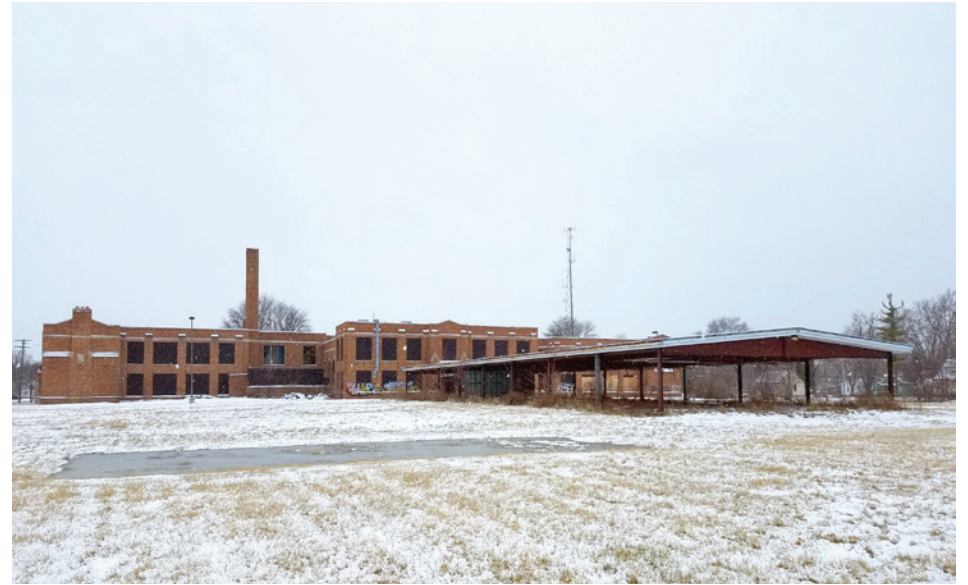
A long prefab classroom wing was added to the rear (north) side of the school. Only the structure and roof remain. This image also shows a portion of the unusually large school yard behind the school.
