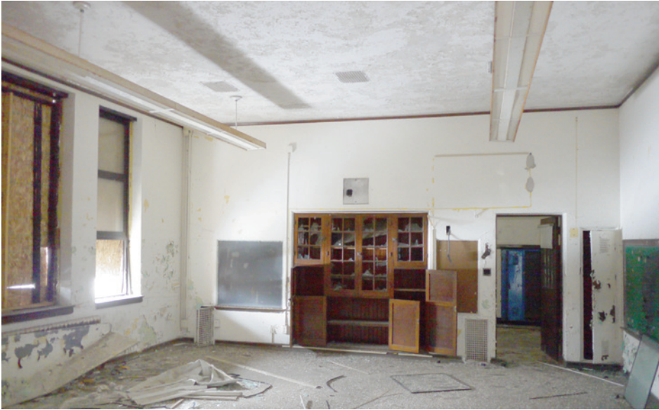
Classrooms in the older north unit feature plaster walls, built-in cabinetry and wood window frames. The original windows were replaced with modern aluminum windows, but many of those have since been scrapped.
