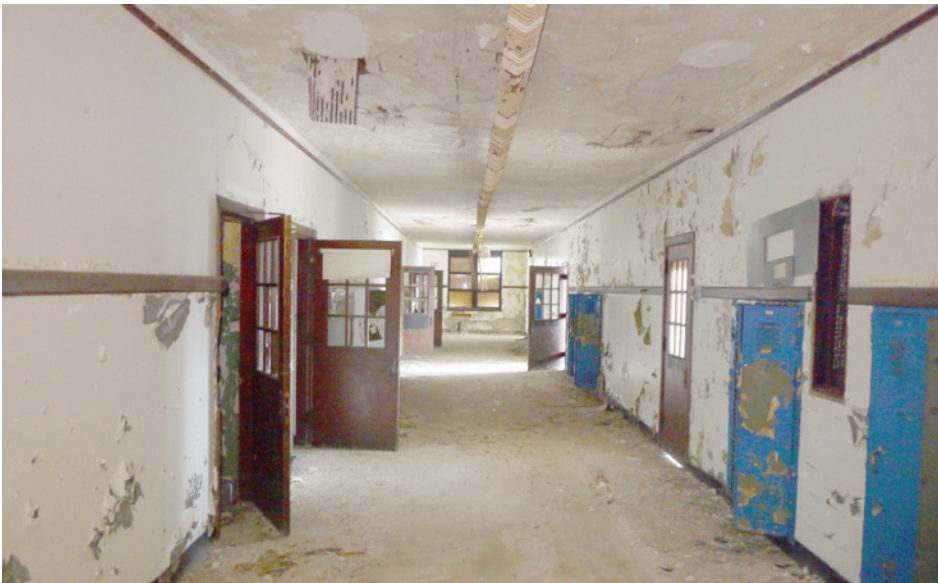
A corridor in the original 1925 wing, with plaster finishes and built-in lockers.
