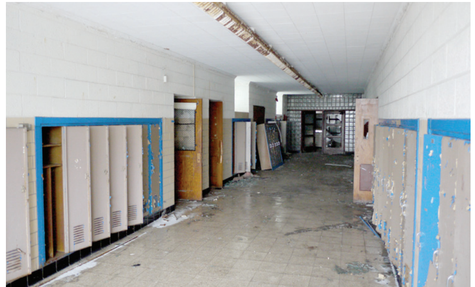
A corridor in the 1951 wing, with painted CMU, glass block, and built-in lockers.
