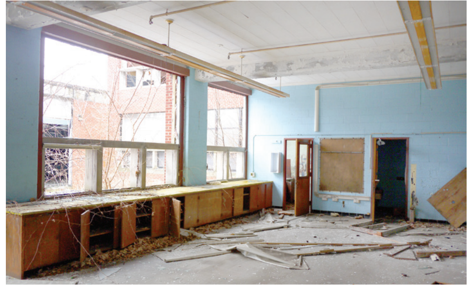
Classrooms in the 1951 addition featured large modern-style windows which formerly held glass block with operable steel-frame lites below. The original materials appear to have been replaced with aluminum frame windows, but those are largely missing.
