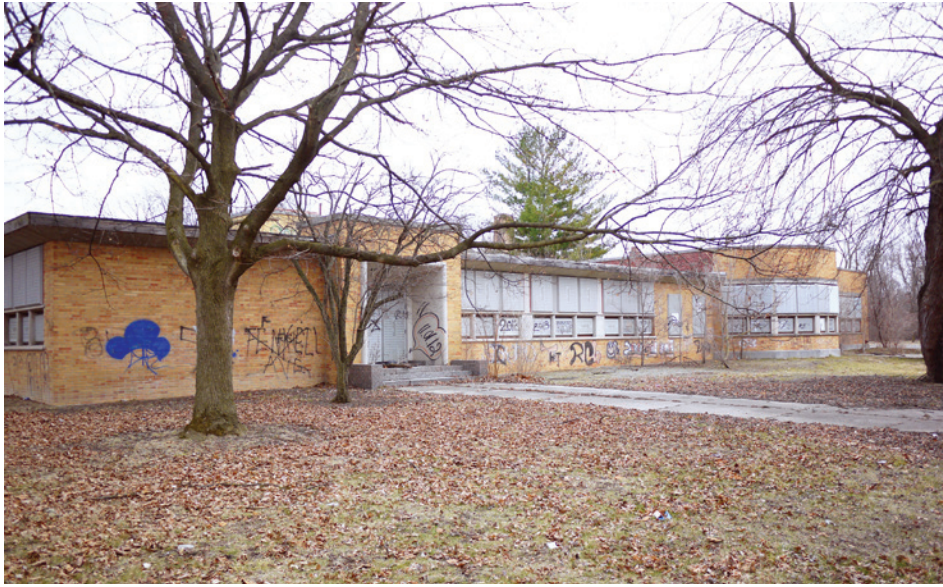
The west facade of the school, showing the original 1924 unit and the 1955 addition. The re-clad original unit includes the large kindergarten bay window and the portion behind it.
