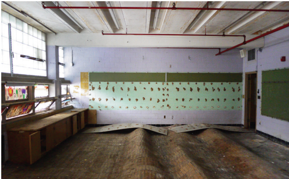
Classrooms are brightly-lit thanks to the wall-to-wall windows. Partition walls can be easily added or demolished thanks to the school's flexible post-and-beam structure.
