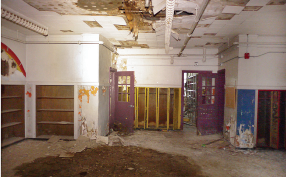
The original unit has four classrooms linked by a cross-shaped circulation/common area. The common space is lined by open cubbies, and feels more like a large room than a corridor.
