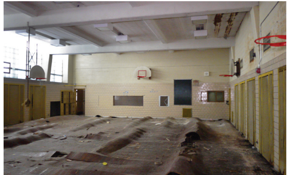
The gym/cafeteria is a 40x60' box with 16.5' ceilings, standard for elementary schools. There is an attached kitchen with small serving window located at the south end (visible on rear wall)
