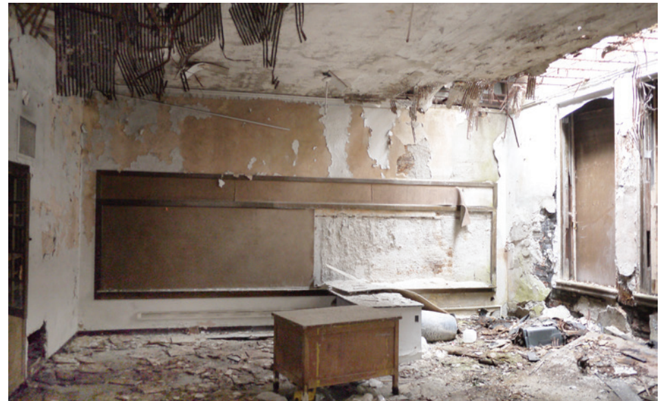
An original 1925 classroom with water damage and partly missing roof. The school building has extensive damage from water infiltration, as well as scrapping and minor fires.
