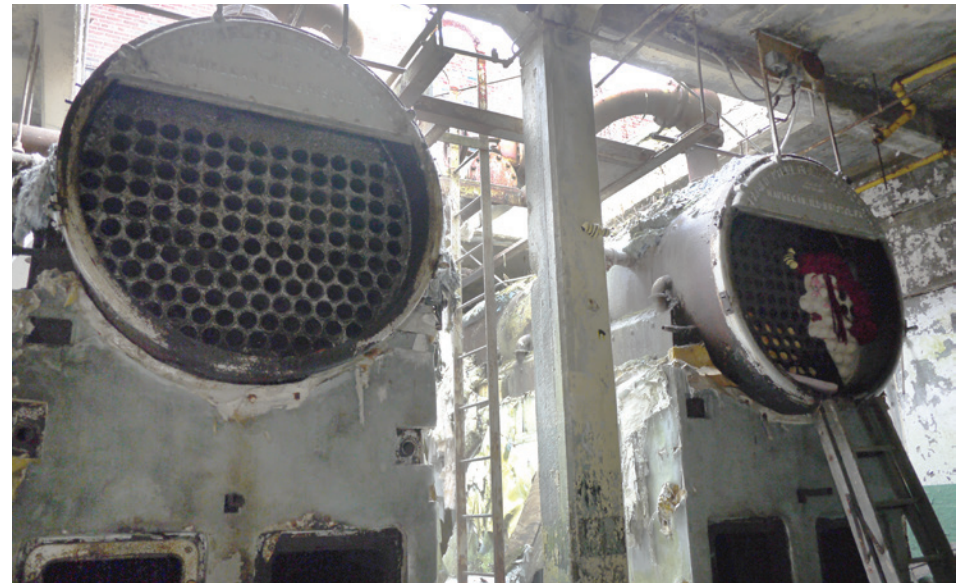
Two massive boilers sit in the pit-like 1930 boiler room. The boiler room is built partly above grade and has an open roof.
