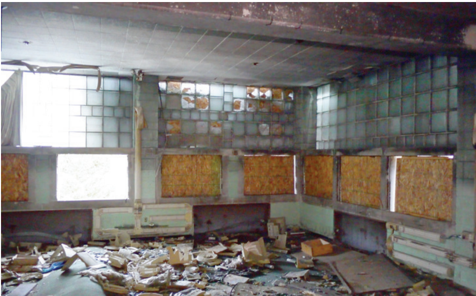
This corner classroom in the 1953 unit displays the modern glass block and steel ribbon windows common of 1950s-era Detroit school buildings.
