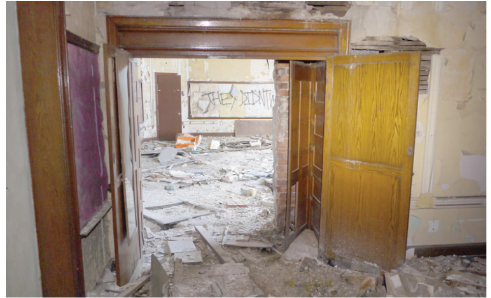
The passage between conjoined classrooms on the second floor reveals the thick walls; inside are brick shafts which travel from the basement through to the attic.
