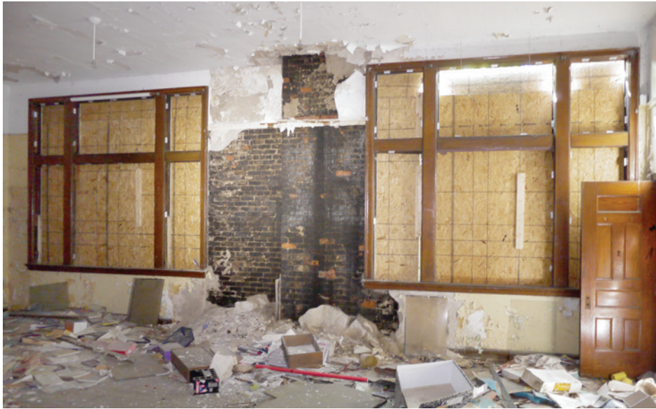
Water damage in an upper-level classroom has caused the plaster walls to disintegrate, revealing the school's load-bearing brick walls. Historic wood window frames are visible, though the original window assemblies and their modern replacements are gone.
