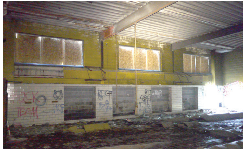
The modern gym/cafeteria is utilitarian steel frame and CMU construction. It has direct exterior access in two locations, but both are below grade and require a short flight of stairs.
