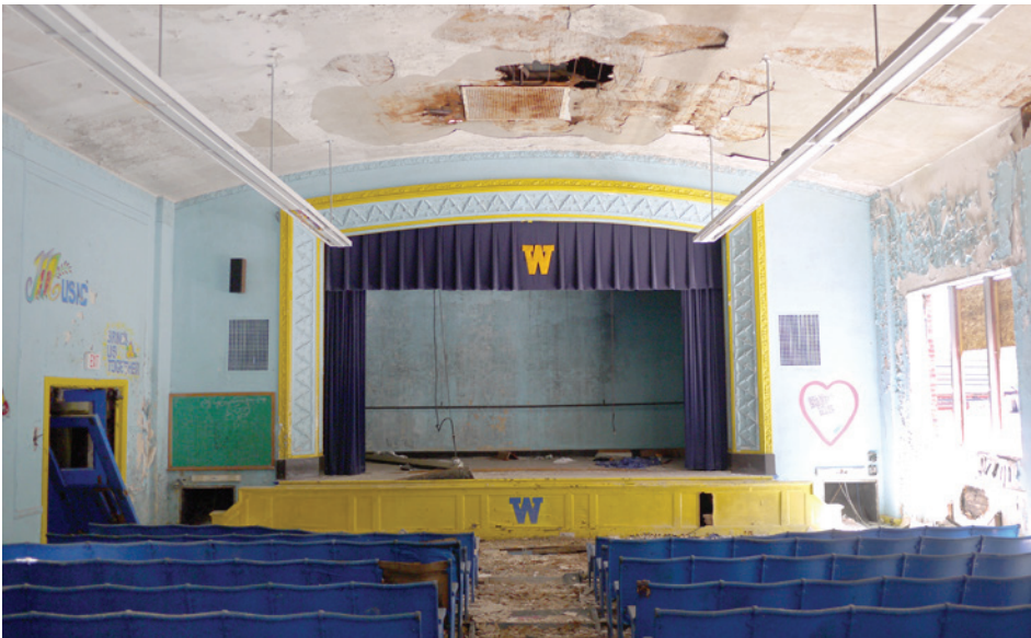
The auditorium has a plaster barrel-vault ceiling and low windows looking into the central lightwell. Water infiltration has damaged the ceiling and wood floors. Seating is still intact.
