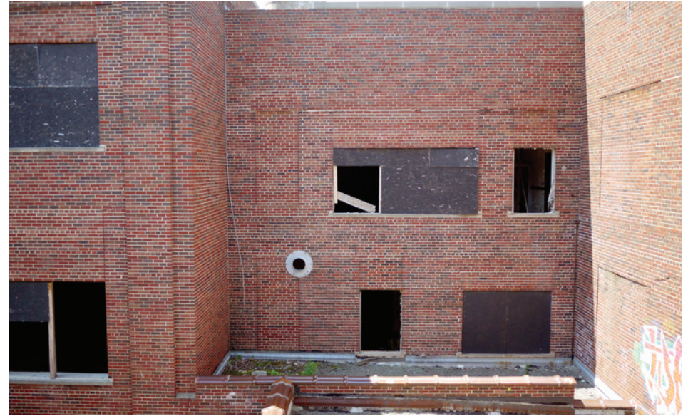
The central courtyard viewed from a restroom. Differences in brickwork show the original location and size of windows. The courtyard allows light and fresh air, but is not accessible. There is also no landscaping or greenery, since the courtyard "ground" is actually the roof of the basement boiler rooms.
