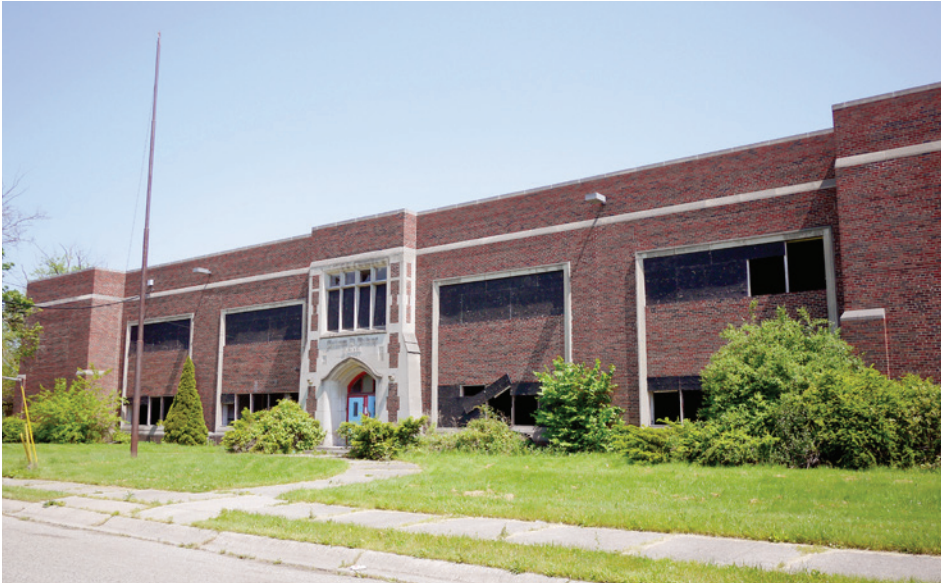
The facade is simple, with little ornamentation beyond the frame-like cast-stone details around the windows and at the parapet. The facade was modified at some point to reduce the classroom windows to horizontal bands.
