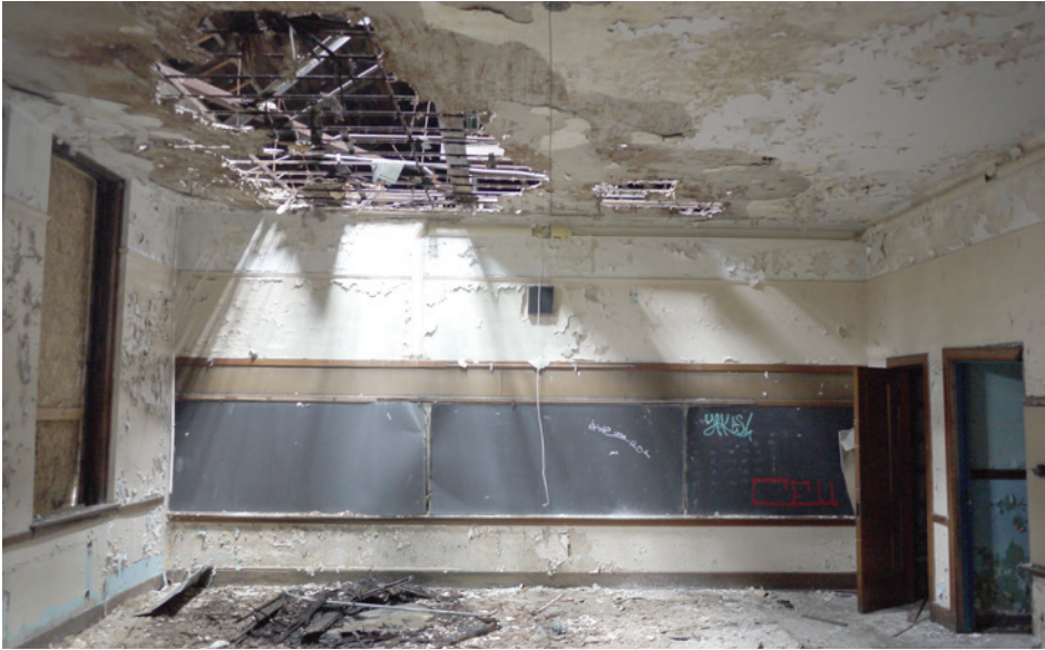
Roof failure visible in a second-story classroom on the south wing. Large openings in the wooden roof deck allow water to infiltrate the wing from top to bottom.
