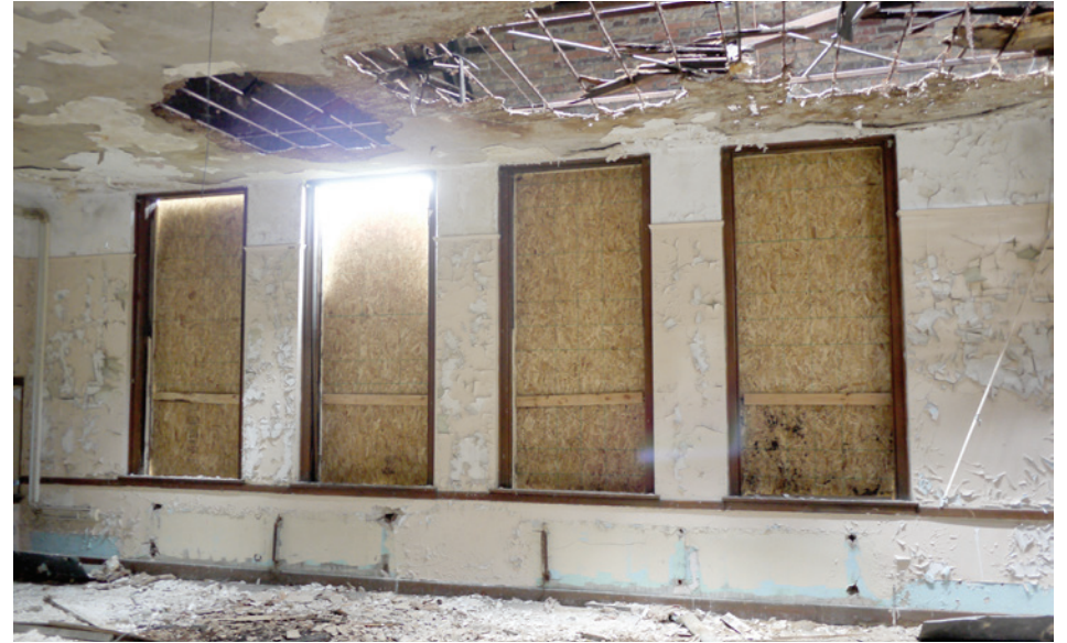
A typical classroom window configuration, featuring four separate wood-framed openings. Windows are scrapped throughout the building.
