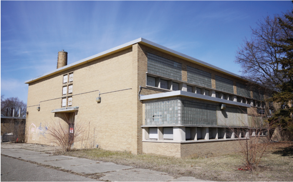
The southeast corner of the building, featuring the 1950s version of the kindergarten bay window. In this version, the traditional 5-sided bay window is replaced by a rectangular glass box.
