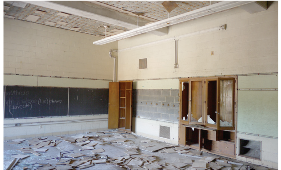
Typical classrooms in the 1946 and 1951 additions are plain, with CMU walls, exposed concrete beams, and extra-high ceilings.
