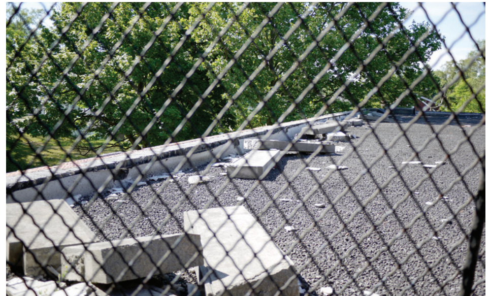
Coping stones pushed onto the roof by scrappers; metal flashing has been taken, leaving wall construction exposed.
