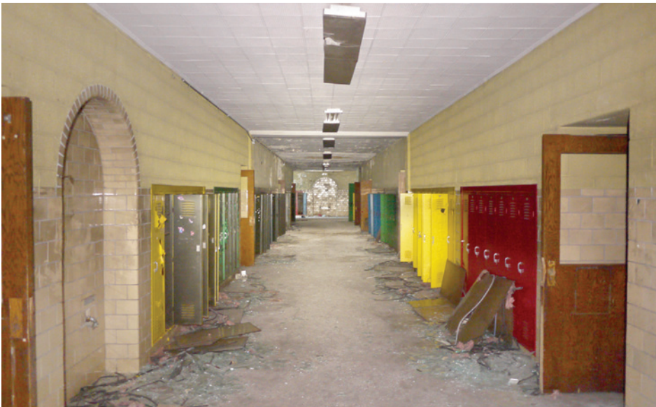
Classroom corridor in excellent condition. CMU and glazed block wall construction with intact lockers and arched drinking fountain alcoves.
