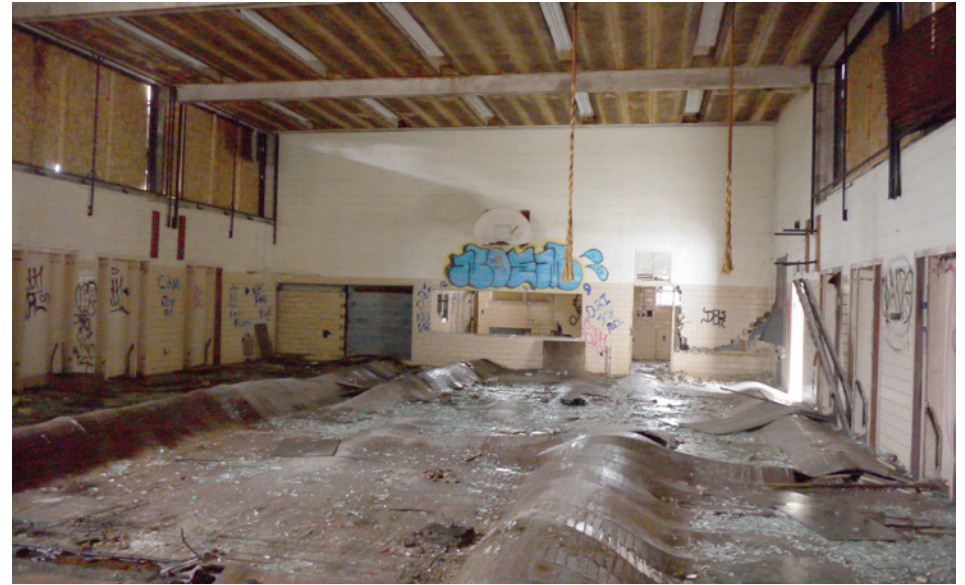
The combination gym and cafeteria is a 40x60' box that features large clerestory windows and 20' ceilings.
