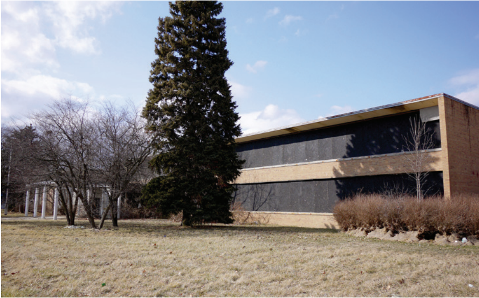
The front elevation viewed from the southeast corner of the building. The main classroom wing is a double-loaded bar featuring continuous glazing along its entire length. The white-columned canopy over the main entrance is visible at the far left.
