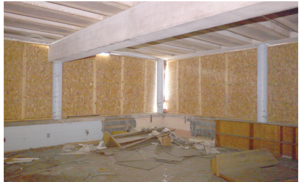
The kindergarten, located at the northeast corner of the building, features continuous glazing on two sides, designed to flood the space with natural light. The school's concrete post and beam structure is clearly visible.
