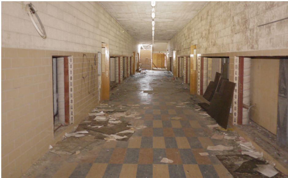
The main corridor on the first floor with lockers removed, but otherwise in good condition. Corridors are 12' wide and double-loaded.
