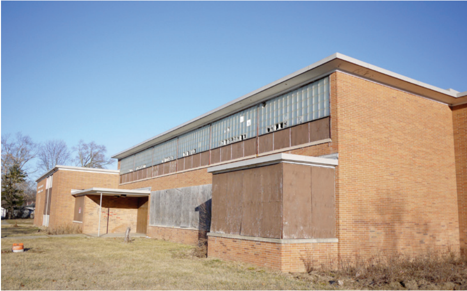
The main (south) facade of the school, showing continuous bands of glass block extending along the entire classroom wing. The windows are largely intact.
