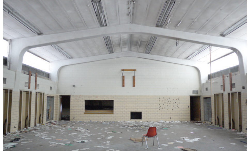
The gym is small but brightly lit, thanks to east and west-facing glass block clerestory windows. The slightly peaked ceiling makes the space feel taller and more open.
