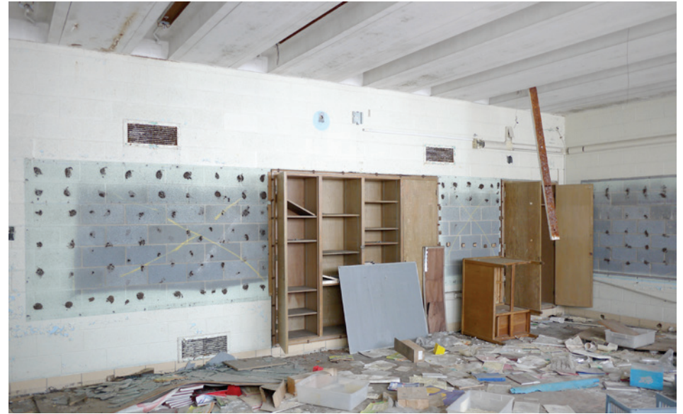
Classroom finishes are simple, including simple wood cabinetry, VCT floors, and an exposed-structure ceiling that incorporates fluorescent tube lights in between the joists.
