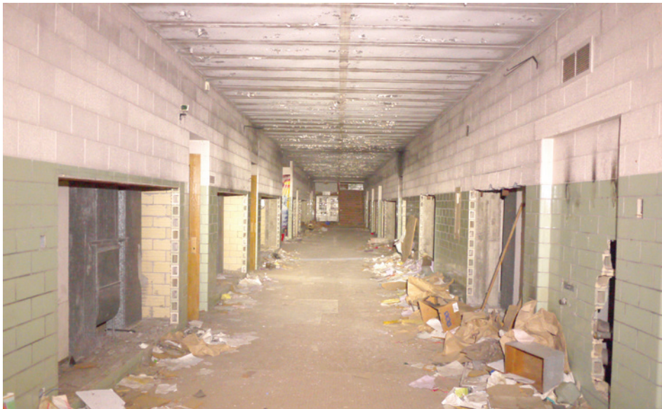
The building has been extensively scrapped, but finishes and structure remain in relatively good condition. The school's corridors feature glazed block finishes with a unique shade of jade green.
