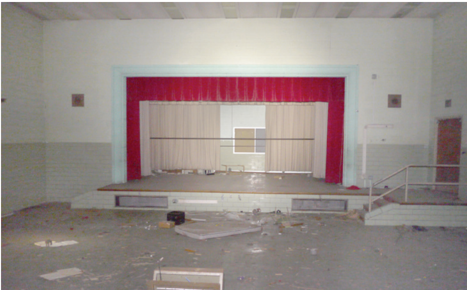
The auditorium is small, with a low stage and a flat sunken floor. The space is a simple box with painted CMU and green glazed tile matching the corridors.
