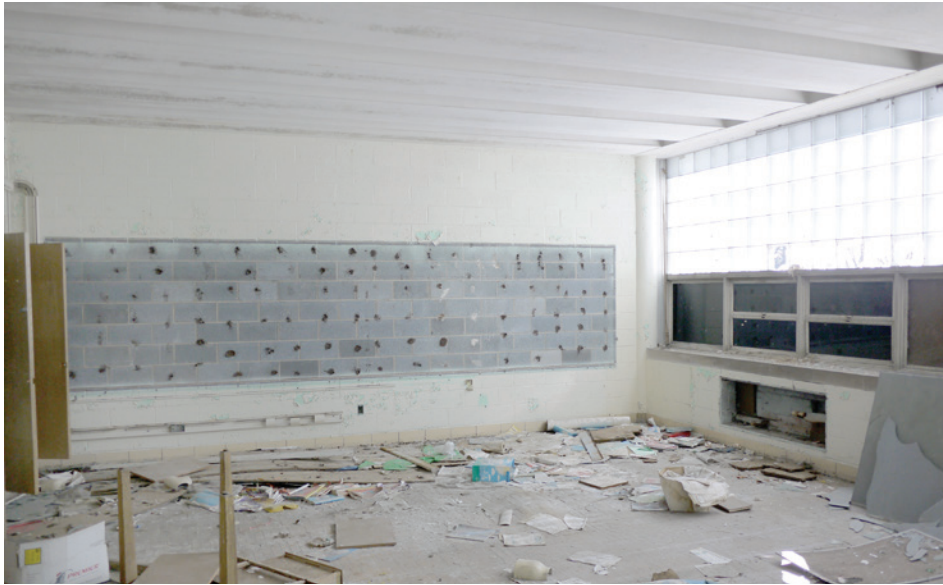
Classrooms are typical of 1950s-era schools, with concrete block construction, and wall-to-wall ribbon windows comprised of glass block over steel-framed operable lites.
