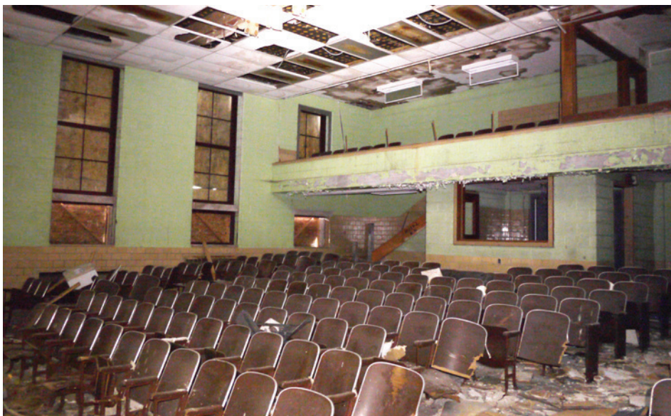
The 1959 auditorium features an enclosed vestibule, a small second-floor balcony, and tall windows on both sides. Finishes are simple, painted CMU block.
