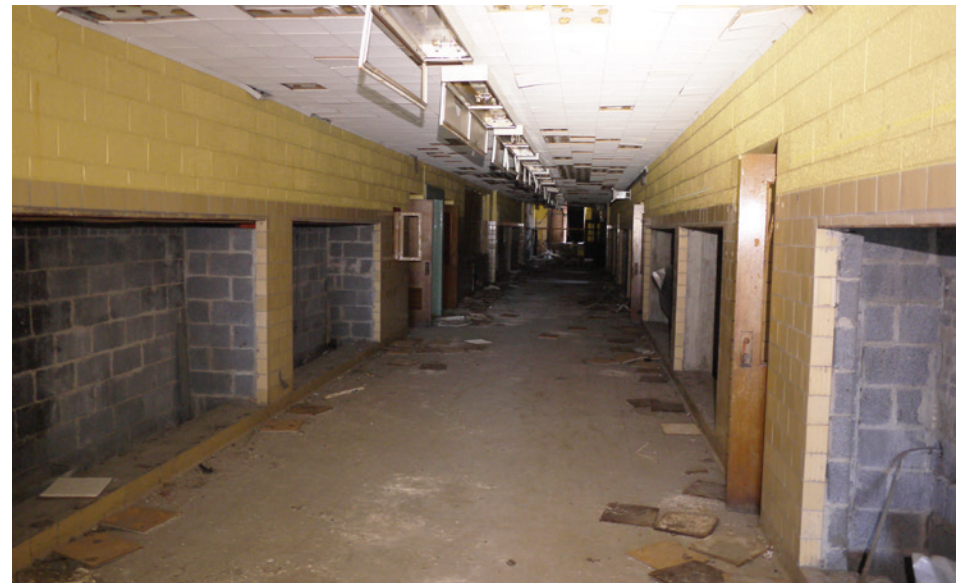
Typical corridor in 1959 addition. Lockers and ductwork have been scrapped, but otherwise the corridor is clean and in serviceable condition.
