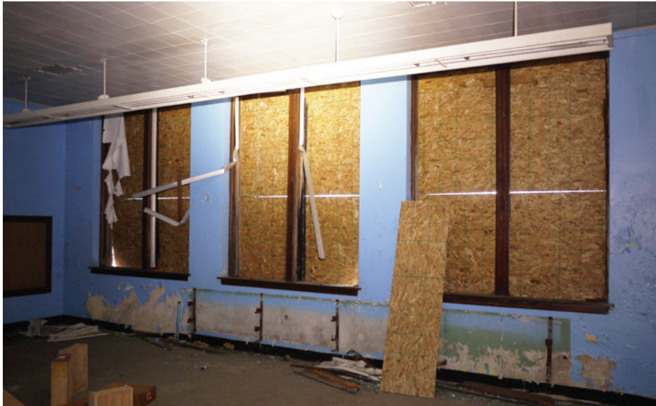
Window configuration and finishes in typical 1925 classroom. Original wood frame windows and their metal replacements are gone; radiators have also been scrapped.
