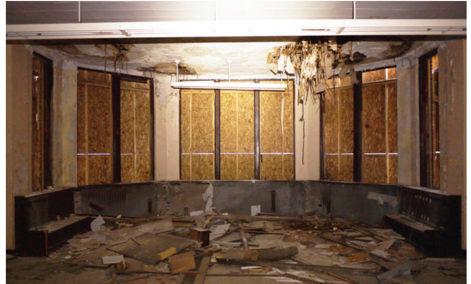
Kindergarten bay window in original 1925 unit. Windows, original wood benches, and radiators have been removed. Water infiltration at the protruding roof has caused plaster failure.
