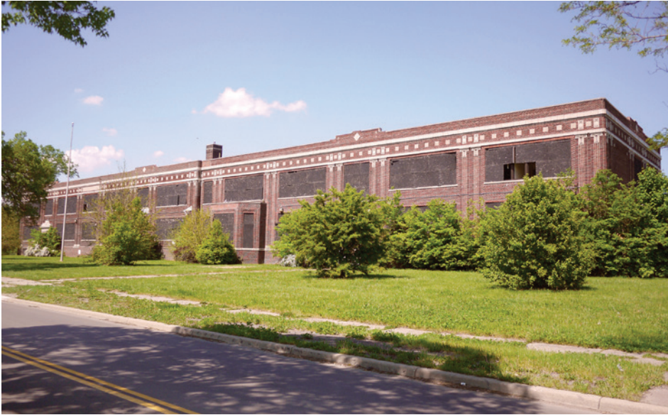
The main/west elevation, with 1923 unit in the foreground, and 1916 unit to the far left of the frame. Although the structural systems of the two wings is different and the two units have different floor heights, care was taken to preserve a unified appearance on the exterior.
