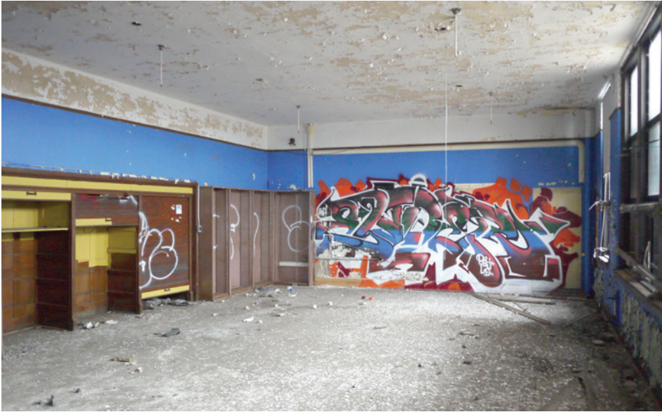
The second floor library is 8' longer than a typical classroom, and features roll-up wood cabinets. Woodwork and walls have been painted over and tagged, but are otherwise in good condition.
