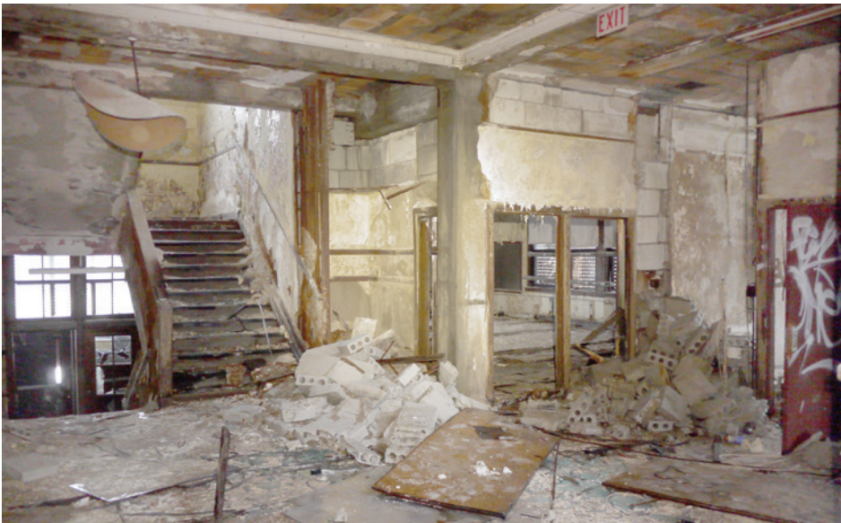
Gypsum block walls on the first floor have collapsed due to water infiltration, revealing the concrete frame. This photo shows the large cross-shaped landing between two facing stairs.
