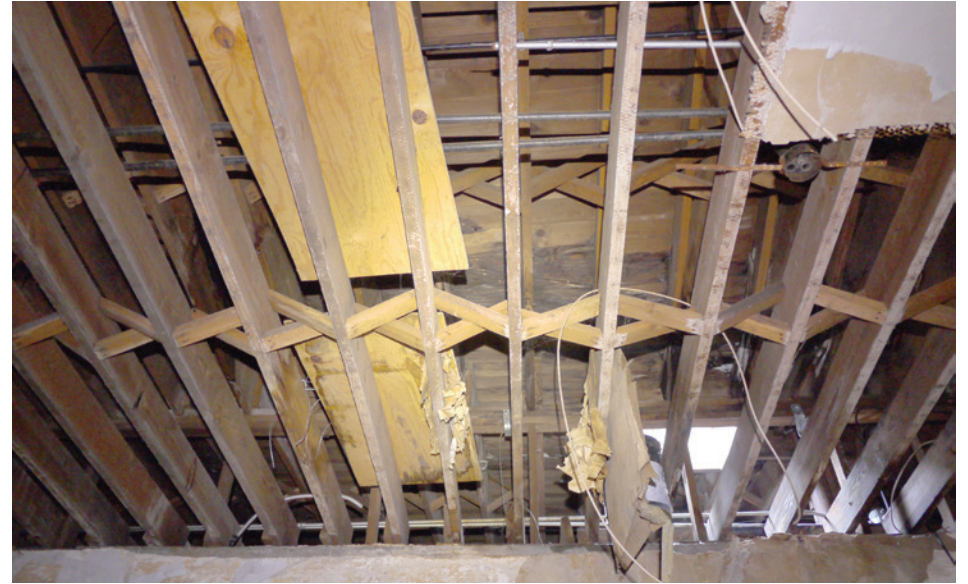
Hanneman has a wood-framed roof sitting on load-bearing brick exterior walls with an internal concrete frame. The roof is water damaged and requires replacement.
